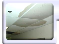
**Roof Leaks:** This is another source of moisture for mold to grow; getting all the areas dried out quickly dosen't give mold a chance to grow.
