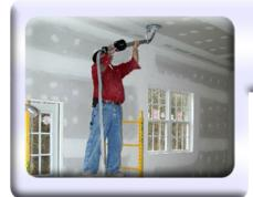
Construction Dust: Can contaminate the HVAC system if it is left running. New construction materials can give off volitile organic compounds, (VOC's) which can be harmful.
